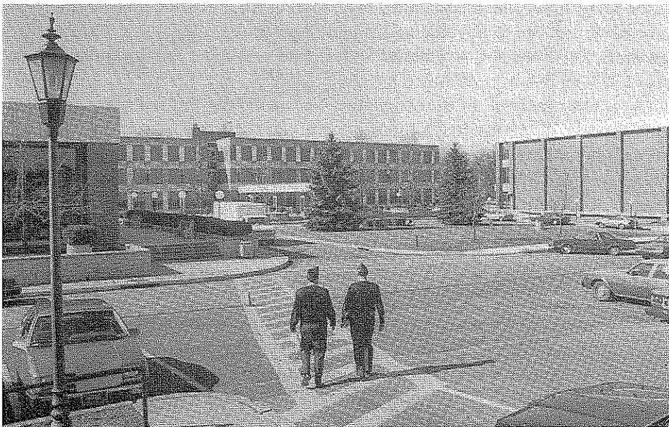
Root Hall (center), home of the US Army War College, at Carlisle Barracks, Pa. Carlisle Barracks was established as a military post in 1757.
